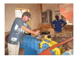
In the Hydro-Electric-Plant of **Kindimba**, which we supported since electrification, the power generation failed after lightning, destroyed the control unit. Bro. Maximilian has installed a new control unit, provided by Licht für Afrika so, that light has come back in time for Christmas.
